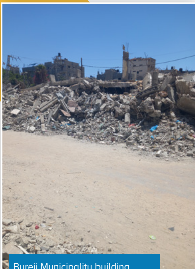
Bureij Municipality building
