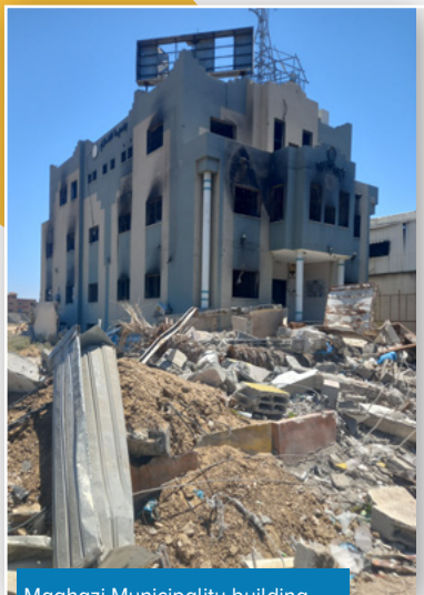
Maghazi Municipality building
